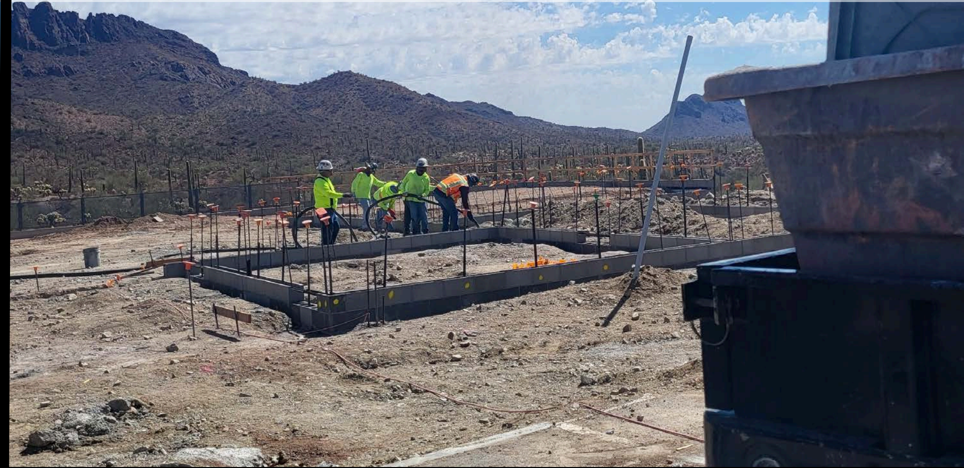
BUILDING STEM WALL FOOTINGS FOR NATURE CENTER
