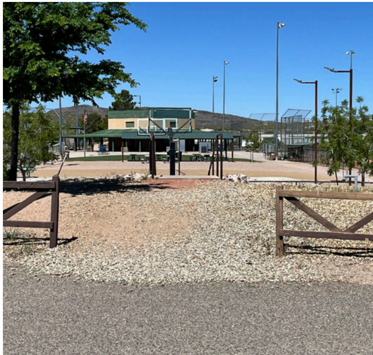
Recommend adding sidewalk to existing stairs. Seal roadways and parking lot throughout and paint light poles throughout.
