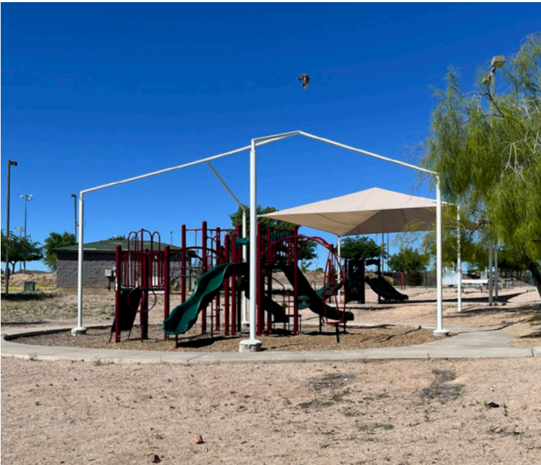
Recommend replacement of playground canopy. Add concrete curb and Fibar fall surface under swings. Replace one swing with ADA accessible swing.
