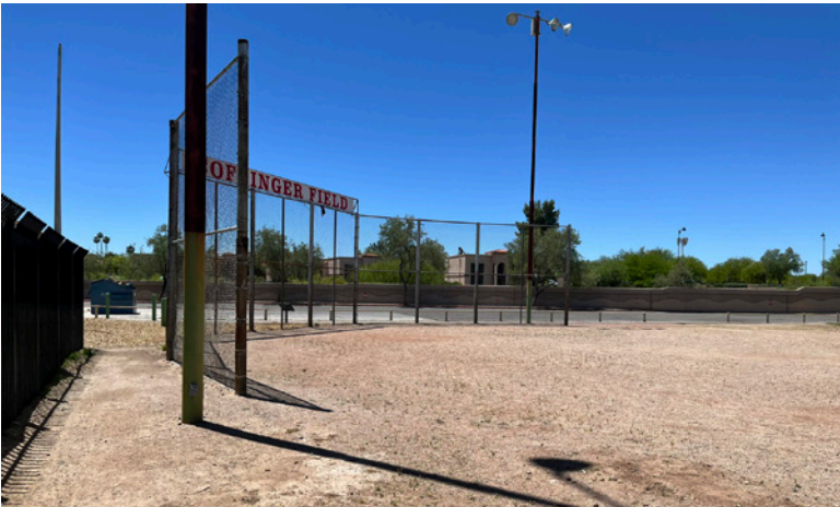
Recommend bringing fields up to programmed field play. Remove and replace infield soil with infield mix, and replace backstop fencing.
