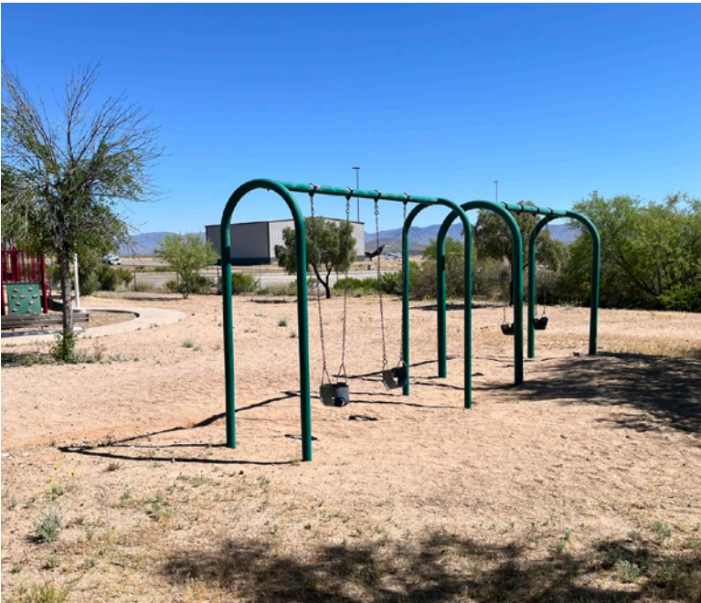
Recommend replacement of playground canopy. Add concrete curb and Fibar fall surface under swings. Replace one swing with ADA accessible swing.
