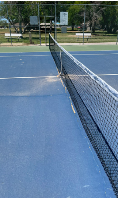
Recommend minor court repair and replacement of court fencing and straightening of posts.
