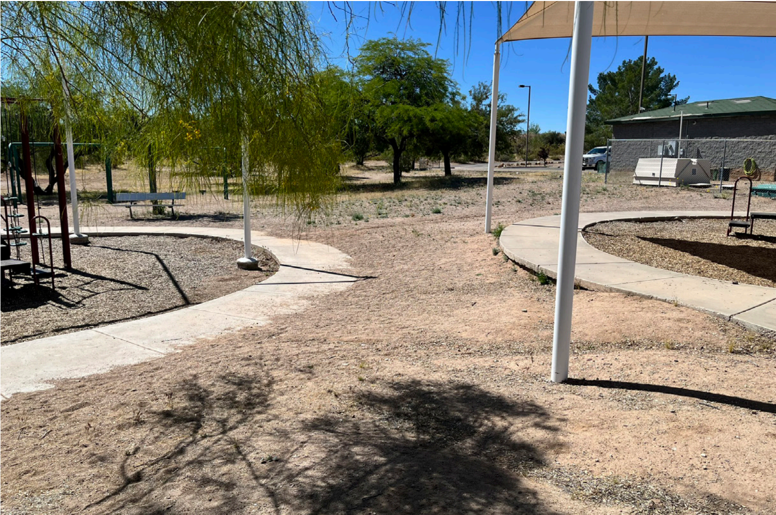
Recommend repairing erosion and adding rock mulch in the ramada and playground area. Add accessible ramps into Fibar play surface.
