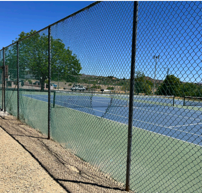
Recommend minor court repair and replacement of court fencing and straightening of posts.
